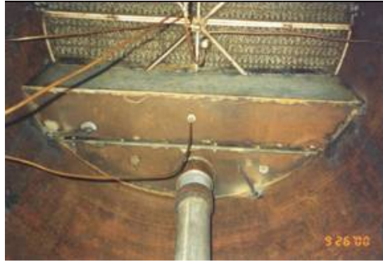
Figure 9. Segmental pan for chordal block test
